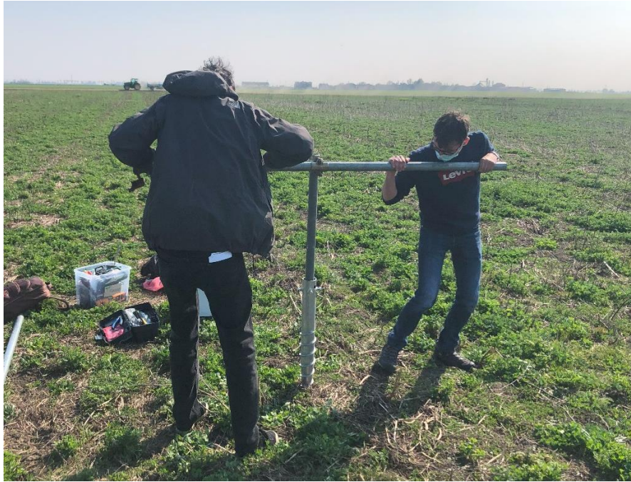
Figure 17 installation of the screw foundation
