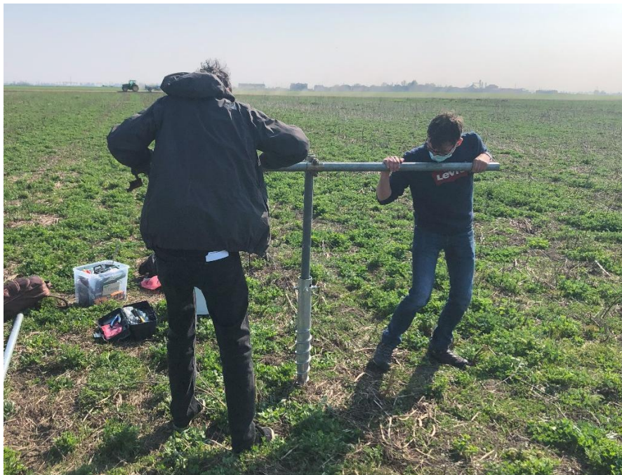
Figure 12: installation of the screw foundation
